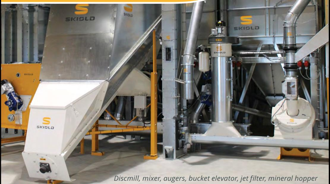
Discmill, mixer, augers, bucket elevator, jet filter, mineral hopper
