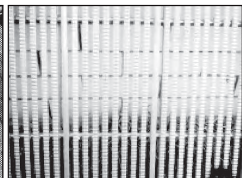
■ Farrowing flooring with a 10mm gap; weaners flooring with a 12mm gap; and growers flooring with a 15mm gap.
